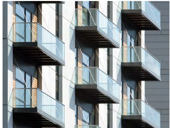
Cantilevered balconies at Residential Units add character, depth, and shadow to the facade
