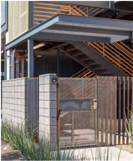
Service Area Screen Wall
