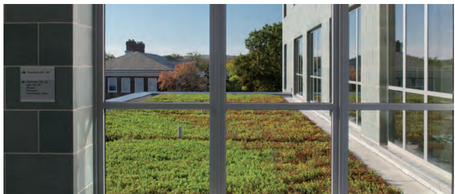
University of Delaware, Science and Engineering Lab
