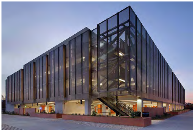
Screened parking structure in Phoenix, AZ.
