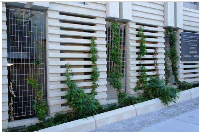
Parking Screen Wall at NY Botanical Gardens
