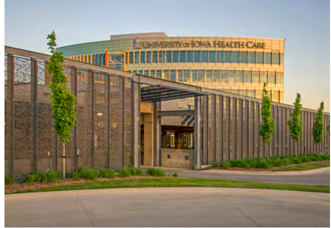
An ornamental perforated metal facade screens a garage.
